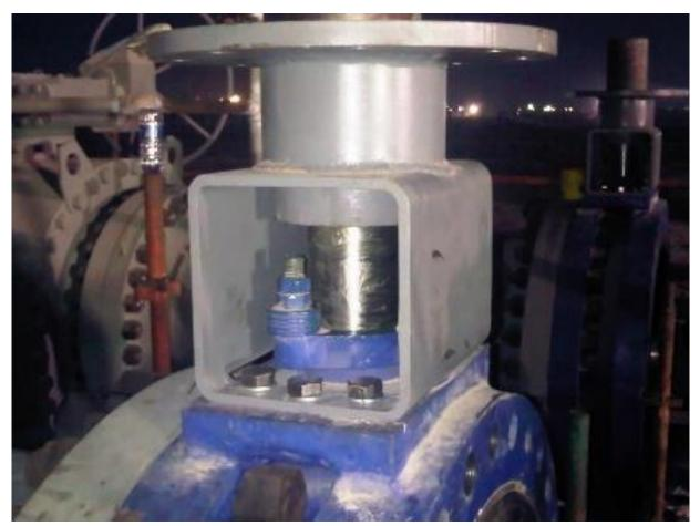
The category of valve determines the sizing procedure. For quarter-turn valves, the torque information has to be gathered from the valve maker or from a reference database at the actuator manufacturer. The torque for multi-turn valves, however, can often be calculated using tried and proven calculation methods available at the actuator manufacturer.
