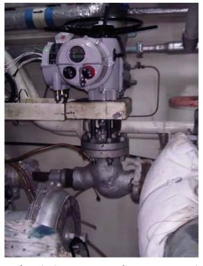
workhours spent manually operating valves. Retrofitted plants can run for an increased number of hours per day, further increasing return in investment and efficiency.
